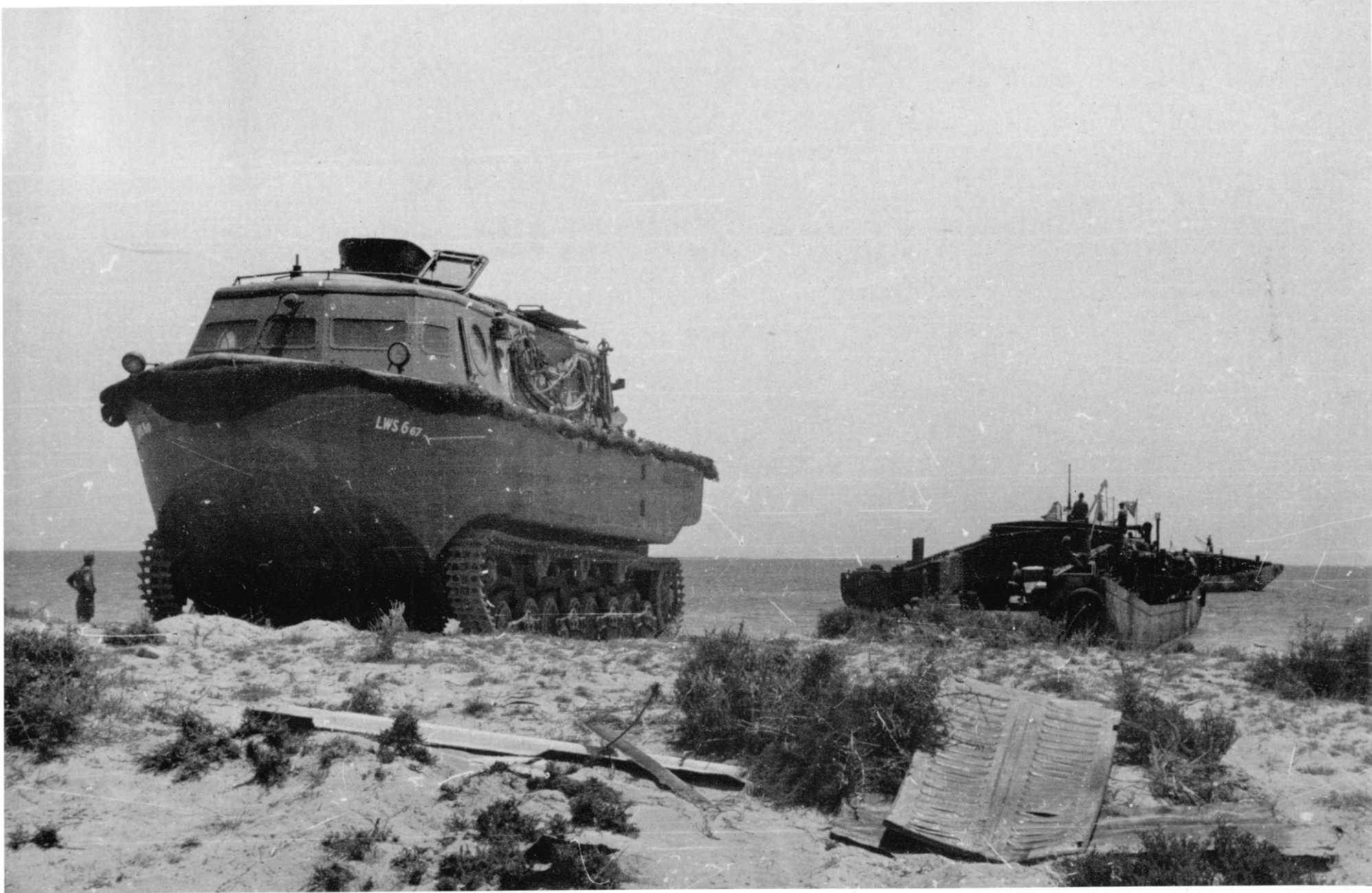
Some of the 21 Land-Wasser-Schlepper were assigned to the shipyard companies of the landing engineer battalions. The vehicles were used primarily in the eastern theater of war, such as in the occupation of the Baltic islands in 1941. The LWS was to be used as a towing tractor on land and a motorized towboat on the water. For these tasks, the vehicles were equipped with a powerful winch. (BA)
